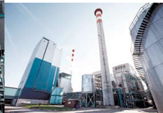
The new ANDRITZ recovery boiler at Cacia (left) replaced two old units (center) and has enabled the mill to expand its production. ▼
