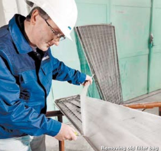
Removing old filter bag
