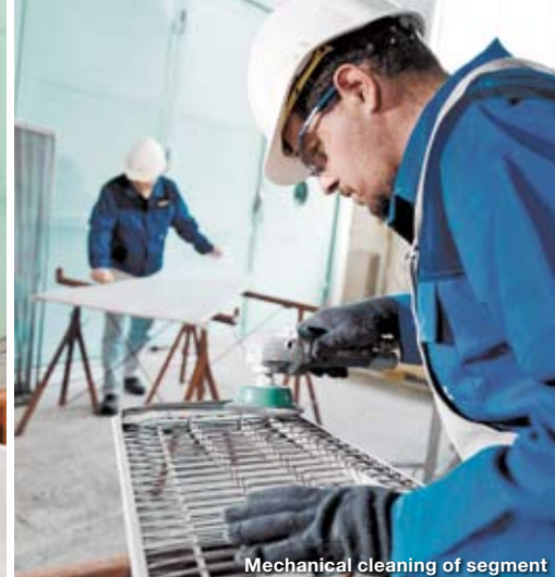
Mechanical cleaning of segment
