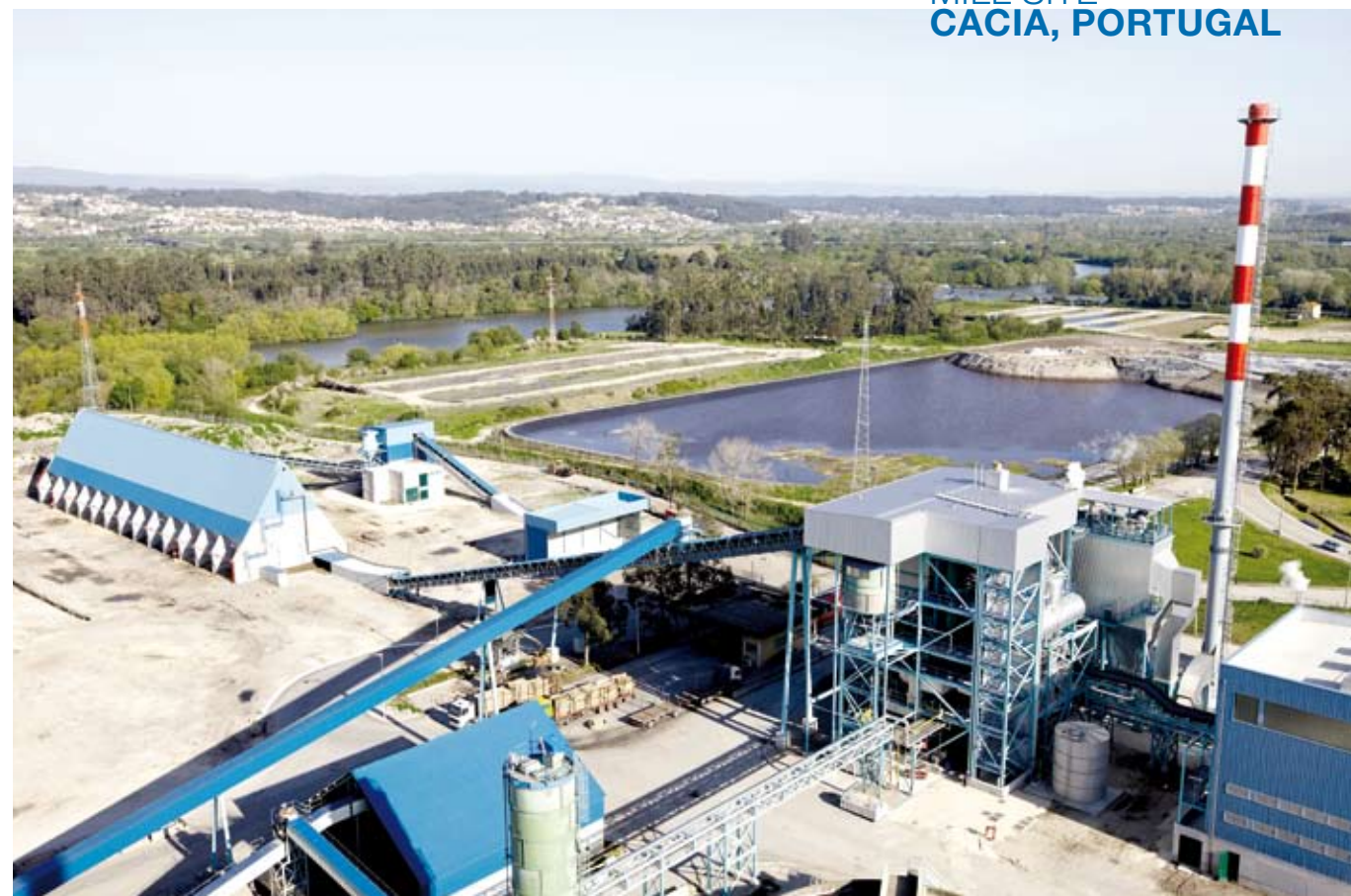
View from above: the ANDRITZ biomass boiler plant at Cacia, with the Vouga River in the background. ▼
