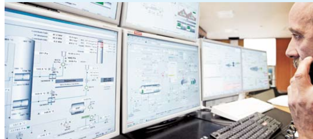
Operator in the Cacia control room. An ANDRITZ service provides remote diagnostics and longer term trend optimization for the biomass boiler. ▼
