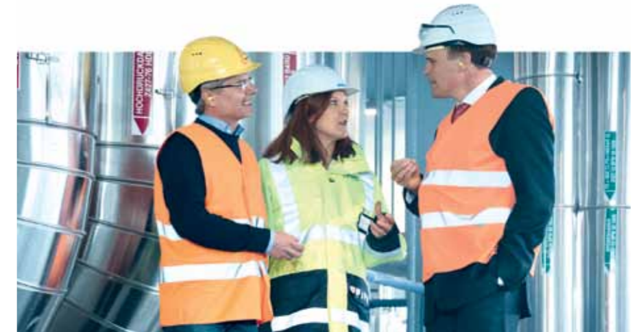
▲ (Left to right): Günter Leitner, Mondi's Technical Manager and Project Manager for RB4; Marja Heinola, Director of Recovery Boiler Sales for ANDRITZ; and Manfred Hacker, Pulp Mill Manager inside the new recovery boiler.
